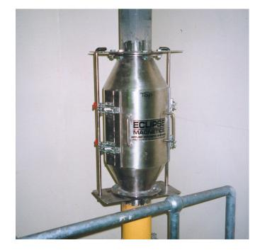
Housed Bullet magnets are ideal for the removal of tramp type contamination, for example nuts, bolts, staples etc., from gravity and pneumatically conveyed pipelines.
